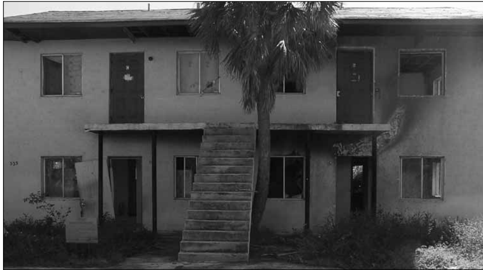
Old vacant apartment in the Riviera Beach Redevelopment Area
