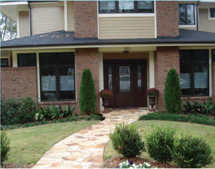
An upscale, barrier-free home by Rawlings Design, Inc. benefits everyone with its accessibility and visitability.
