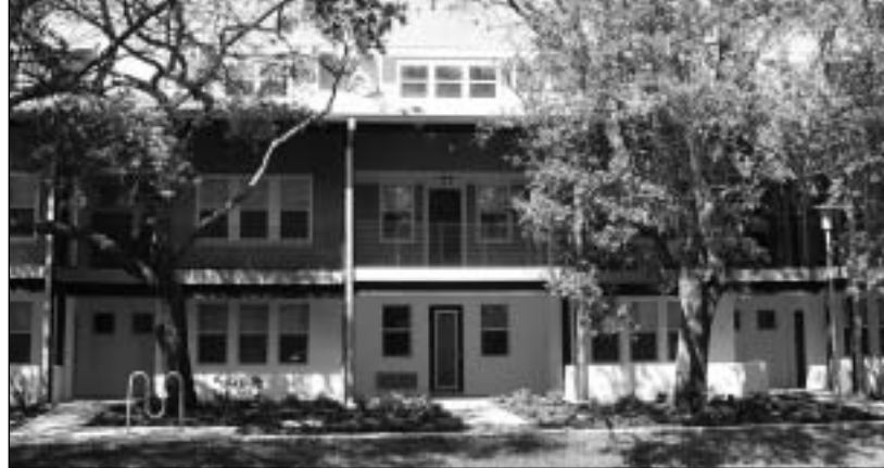
Over 30 percent of surfaces are shaded. Large covered roof overhangs that reduce solar gain. Energy efficient inate glass operable windows.
