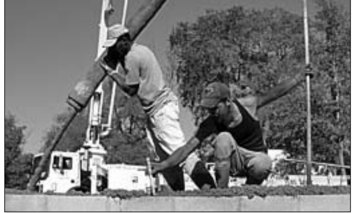
The foundational slab was made partially from recycled concrete.
