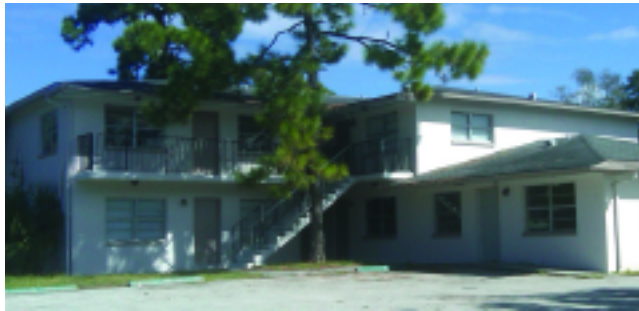
A seven unit apartment complex purchased by the City of Ft. Myers. Once rehabilitated it will be deeded to a nonprofit supportive housing provider for families who are rebuilding their lives after foreclosure, evictions, homelessness and unemployment. Support services include education and training for new careers.
