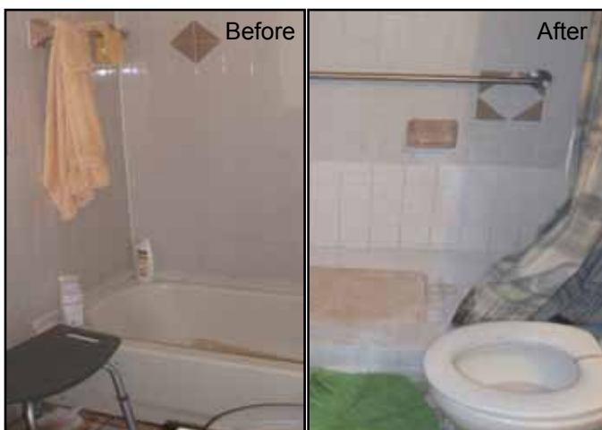
Before and after photos of bathroom repairs financed with SHIP.
