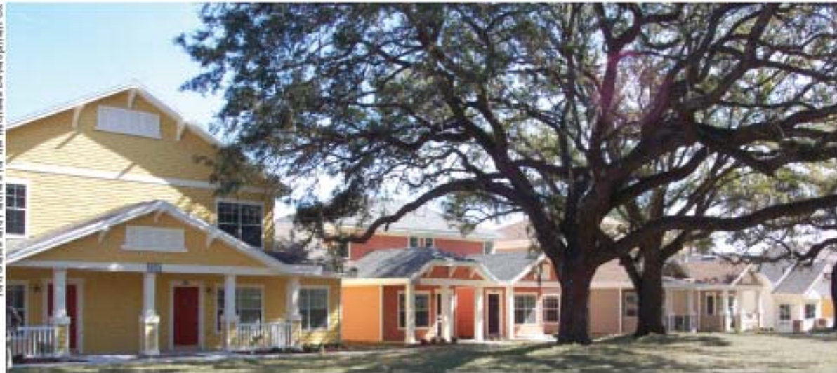
"Airplane" and "Camel Back" style duplexes are two of the designs The Michaels Development Co. (Torti Gallas and Partners, used in Belmont Heights Estates, an affordable housing development in Tampa built with a variety of funds including multi-family bond financing from the Hillsborough County HFA.
