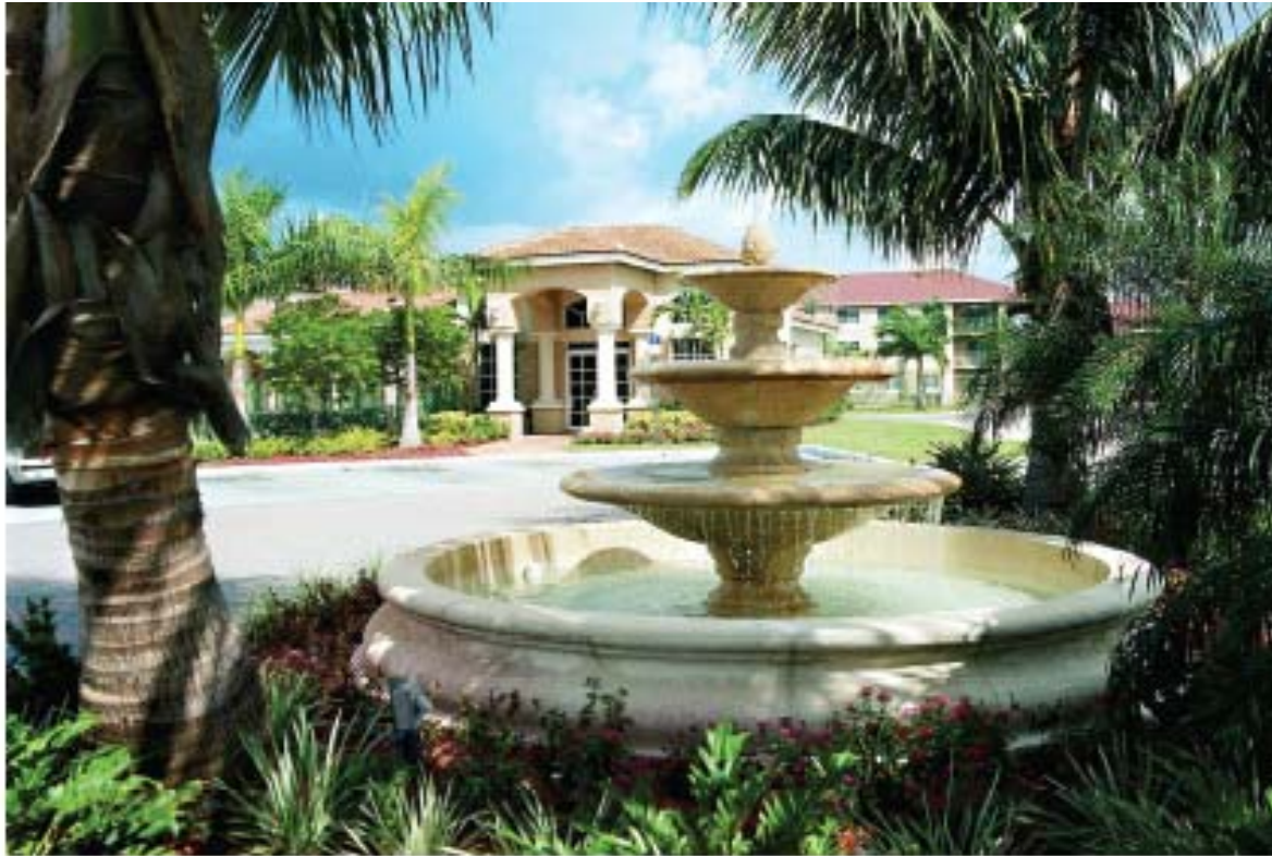
The Crossings is a 320 unit community in Miami, financed with $13.5 million in tax-exempt bonds issued by the FHFC. One hundred percent of the community is set aside for residents earning less than 60% of the area median income. The oversized 5,000+/- sq.ft. clubhouse depicted here, includes a community/social room for a variety of resident programs and amenities including a kitchen in which Otis Spunkmeyer cookies are baked throughout the day.
